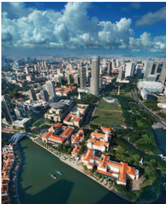
Singapore – growing on sand imported from beyond its national borders. The country's surface area has expanded by 22% since the 1960s
